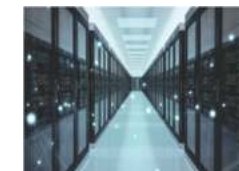
Small and medium-sized data center
